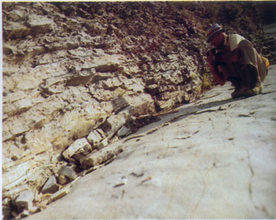
Location 18-9, below western third of headscarp; outcrop along edge of failure surface of 1963 slide or post-1963 slides; loose rock slabs cover clay interbed with dip of 35°
